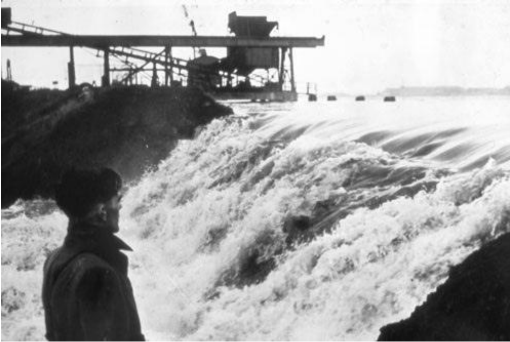
A breach at Erith after the North Sea flood of 1953
