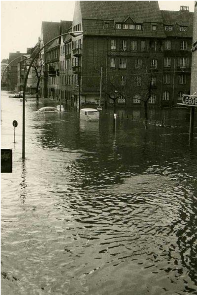
Flooded crossroad in Wilhelmsburg, 1962
