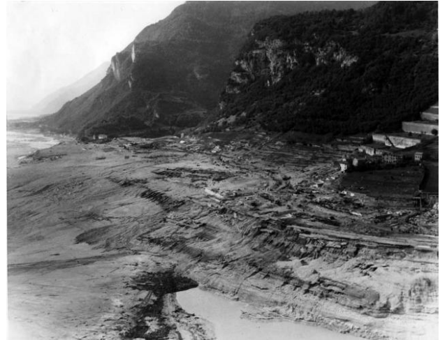
View of Longarone after the wave from the Vajont Dam (1963).
